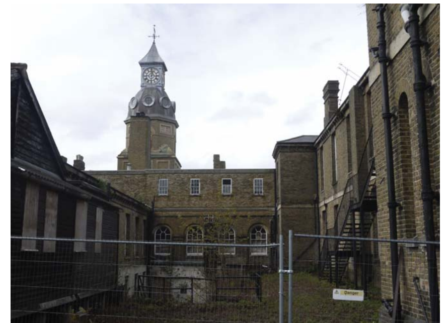
Current state of the central rear courtyard
