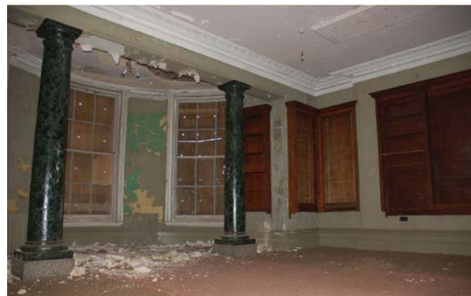
CMH - Internal condition of the Administration block
