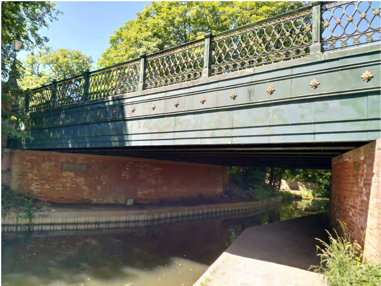
Image 19— View South West of the locally listed Iron Bridge
