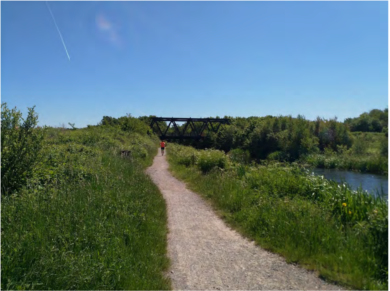
Image 5—View looking West towards Eelmoor Bridge
