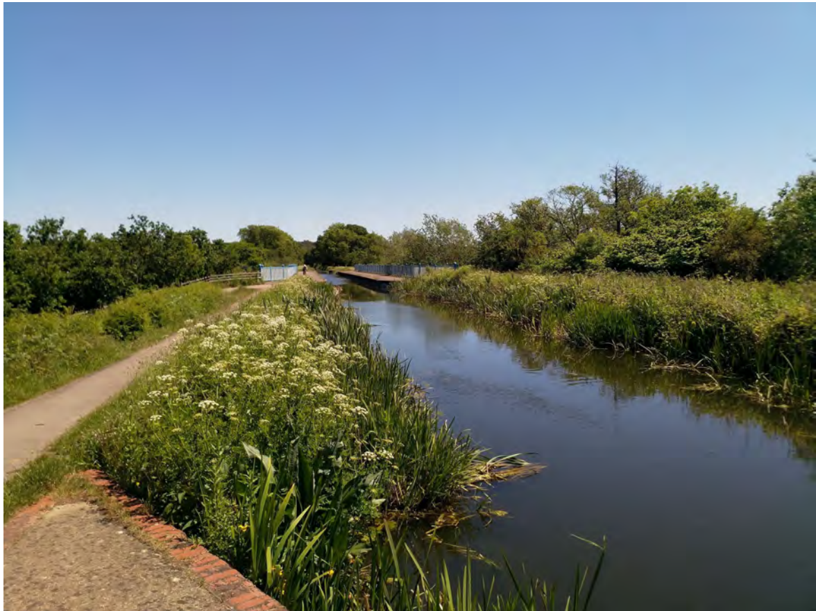
Image 29— View looking east towards the aqueduct over the Blackwater Valley Road
