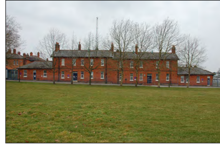
6. Military Police Barracks. Built in 1898 as Military Police Barracks and stables. Currently used as offices for the Royal Logistics Corps. Curtilage and locally listed.
