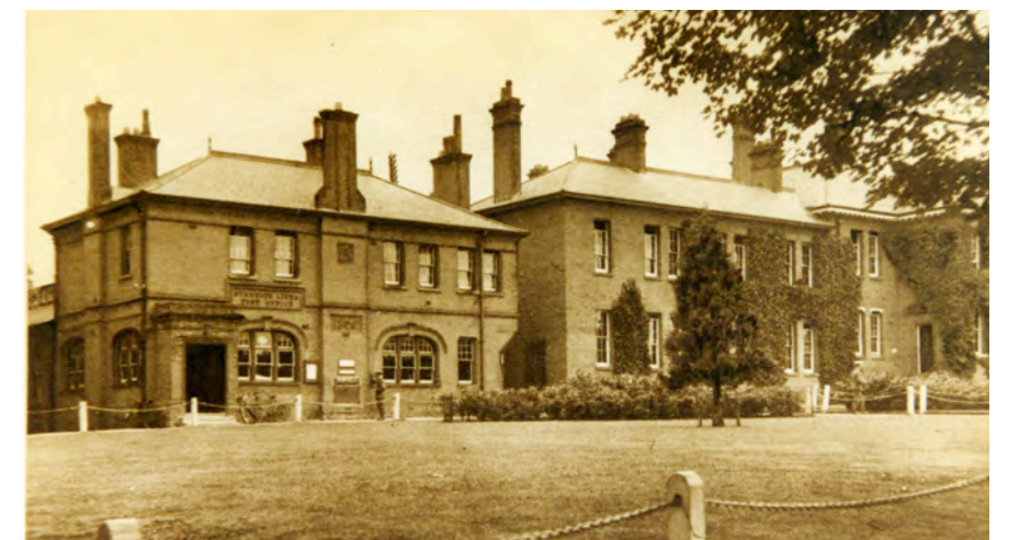
The Old Post Office fronting onto Queen's Avenue
