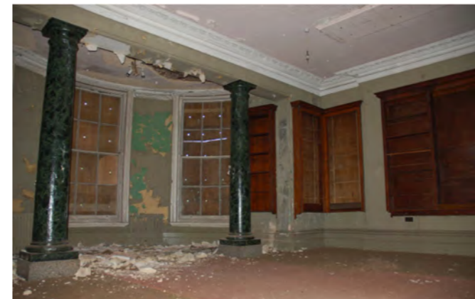
CMH - Internal condition of the Administration block
