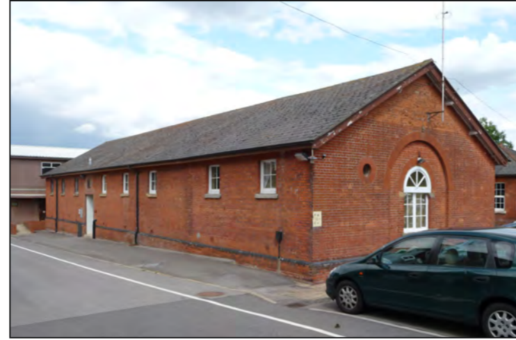
5. Stable Block. Built in the 1890's as military stables. Subdivided in recent years to form a conference room, gymnasium and store.
