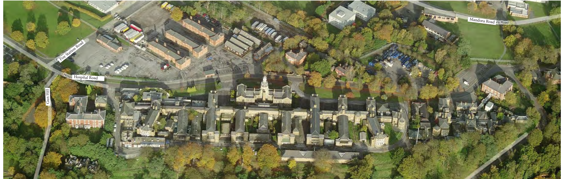
Cambridge Military Hospital, which comprises the Grade II -Listed CMH, Louise Margaret Hospital, McGrigor Barracks and various other buildings
