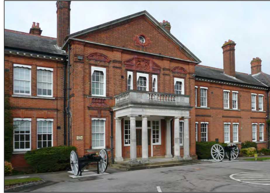
1. Former 4th Division Headquarters building. Purpose-built as a headquarters building in 1894. Grade II Listed. Brickwork detailing and main internal staircase are particularly fine. The plan form is U-shaped, enclosing several outbuildings in a rear courtyard. Internally the building is arranged on two floors as cellular offices with corridor access throughout.
