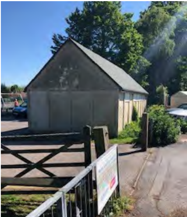
Image 9 —View of modern structure
