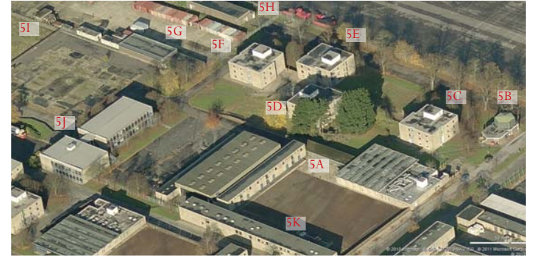
Aerial view of 5 - Normandy Barracks
