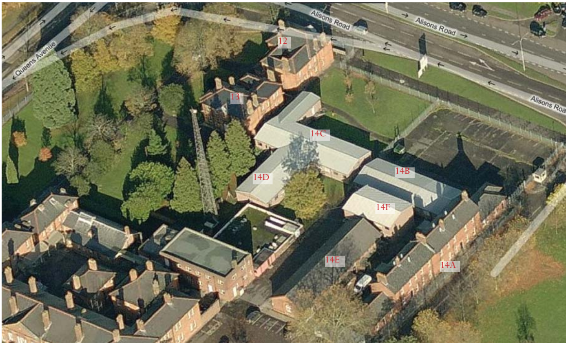
Aerial View of L1 and 12-14 - SE District Headquarters with Alisons House, Cranbrook house Barracks and Stables HQ Division
