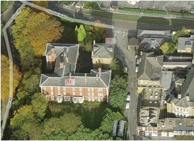
Aerial View of 19 and 20 - Gunhill House and Water Tower
