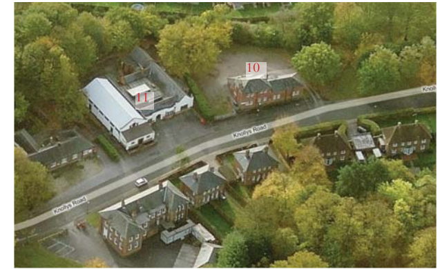
Aerial View of 10 and 11 - Cab Stand and Parcel offices and Civil Service Club
