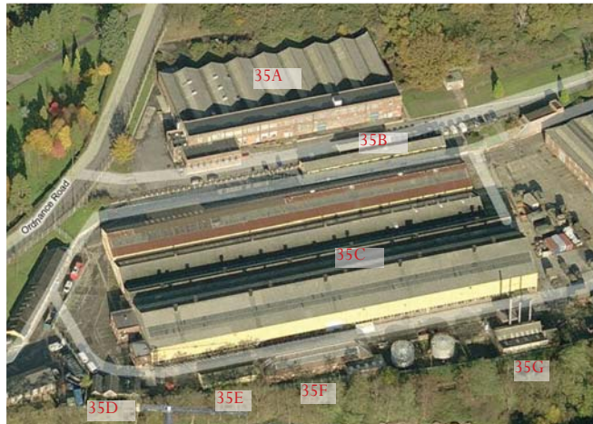
Aerial View of 35- Existing Buildings on proposed HWRC site
