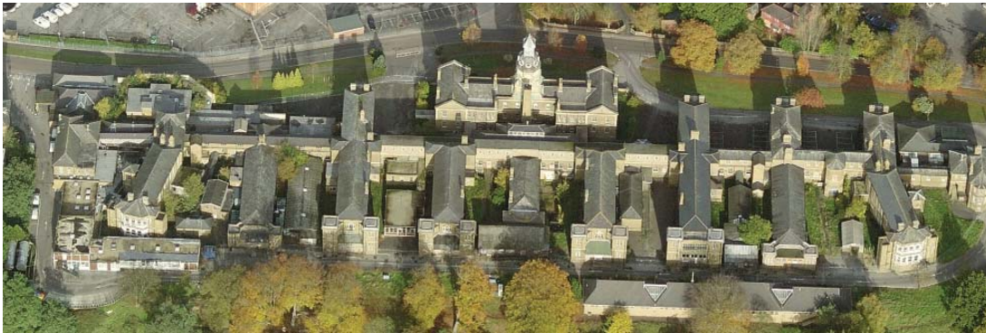
Aerial View of L 5 - Cambridge Military Hospital
