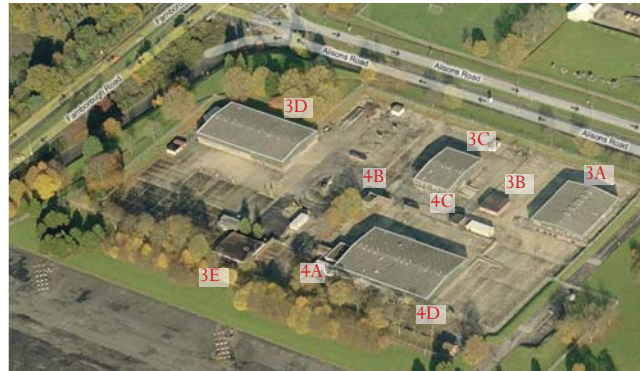
Aerial View of 3 and 4 - Depot and Admin Block
