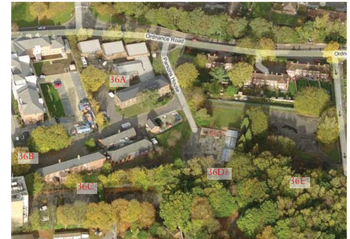
Aerial View of 36 - Existing Buildings on southern most parcel of site
