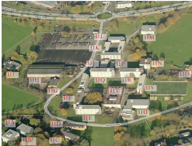
Aerial View of 31 - Buller Barracks
