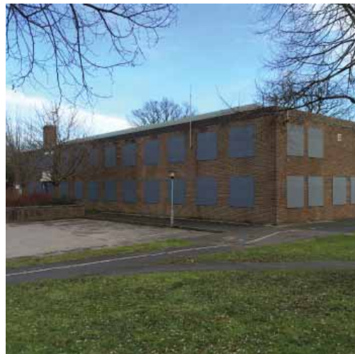
The boarded-up Police Station building
