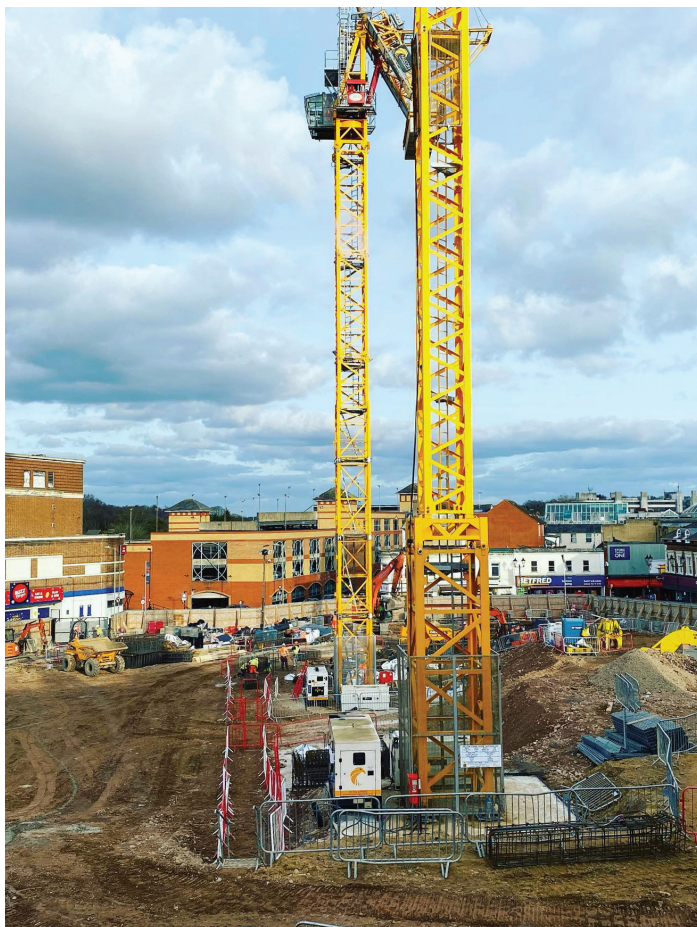
Construction on the Union Yard site, Aldershot town centre
