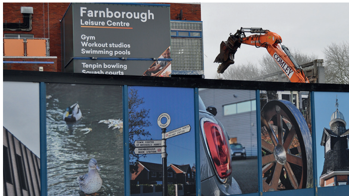
Demolition of the leisure centre, Farnborough
