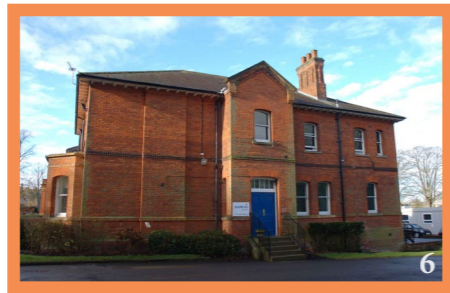
POSITIVE: The side, eastern elevation of the Mandora Officers Mess (28B) is also attractive.
