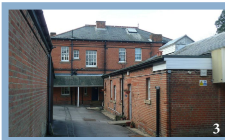
NEGATIVE: Later additions in the area behind the headquarters obscure views and block the courtyard.
