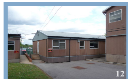
NEGATIVE: Building 14B is similarly unattractive and its removal would open up view to listed building L1.
