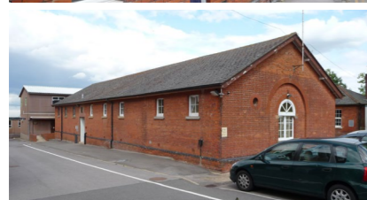
Top: View of the Military Police Barracks (14A), above: the Stable Block (14E).
