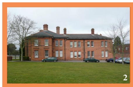
POSITIVE: The side (east) elevation of the main Headquarters building (L1) also retains its original appearance.
