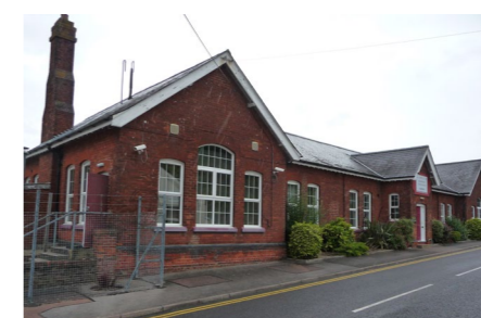
The Gallwey Road elevation of the Signaling School (29F).
