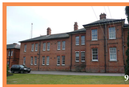
POSITIVE: The western facade of the Headquarters Building (L1) is similarly well preserved.
