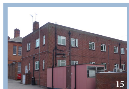
NEGATIVE: Building 14D is a poor quality modern structure that blocks views towards the listed building L1.
