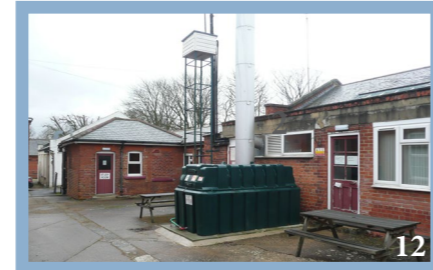
NEGATIVE: However, the rear section of the signalling school is poor quality and littered with modern additions.
