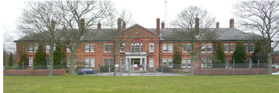
The main facade of the Head Quarters 4th Division (L1)
