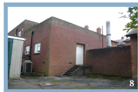
NEGATIVE: Building 14D is a poor quality modern structure that blocks views towards the listed building L1.
