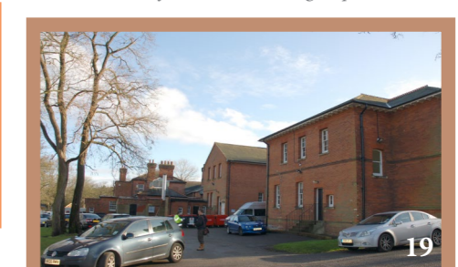
NEUTRAL: The rear (north) elevation of the Mandora officers mess (28B) has many modern alterations which detract from the listed building.
