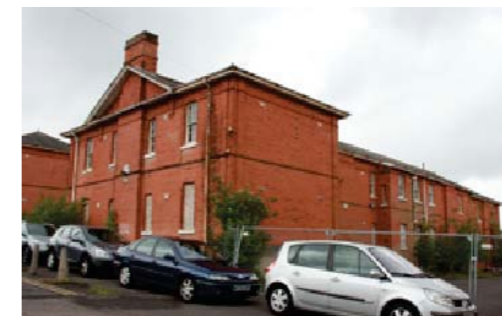
North-west elevation of the Mcgrigor Barracks (16C)
