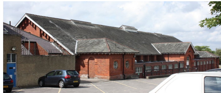
Left: The eastern elevation of the Maida Gymnasium (L3).
