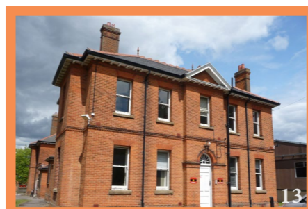
POSITIVE: The southern facade of Cranbook House (13) is a particularly attractive composition.
