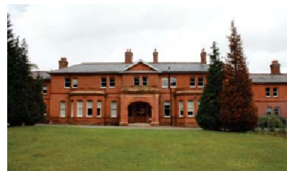
Top: The north elevation of the Mandora Officer's Mess (18B) Above: the south elevation.
