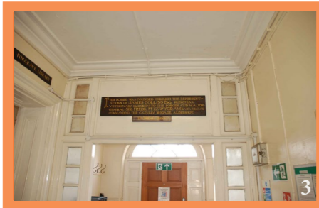
POSITIVE: The interior of Fitzwygram House is relatively intact, and includes a memorial plaque.
