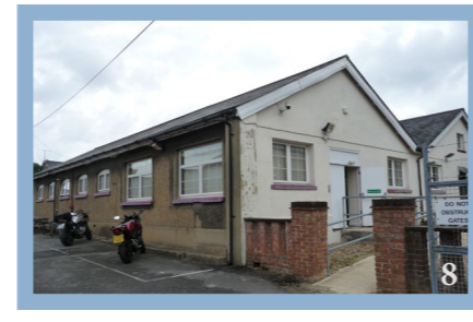
NEGATIVE: Modern utilitarian buildings (29E) facing onto Gallwey Road.
