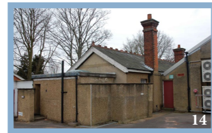
NEGATIVE: The eastern and southern facades of the Vaccine Institute building (29I) are entirely surrounded by modern extensions.
