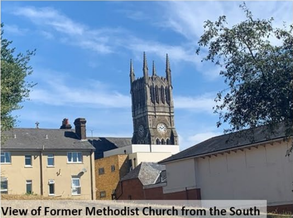
View of Former Methodist Church from the South
