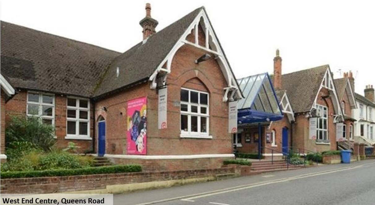
West End Centre, Queens Road
