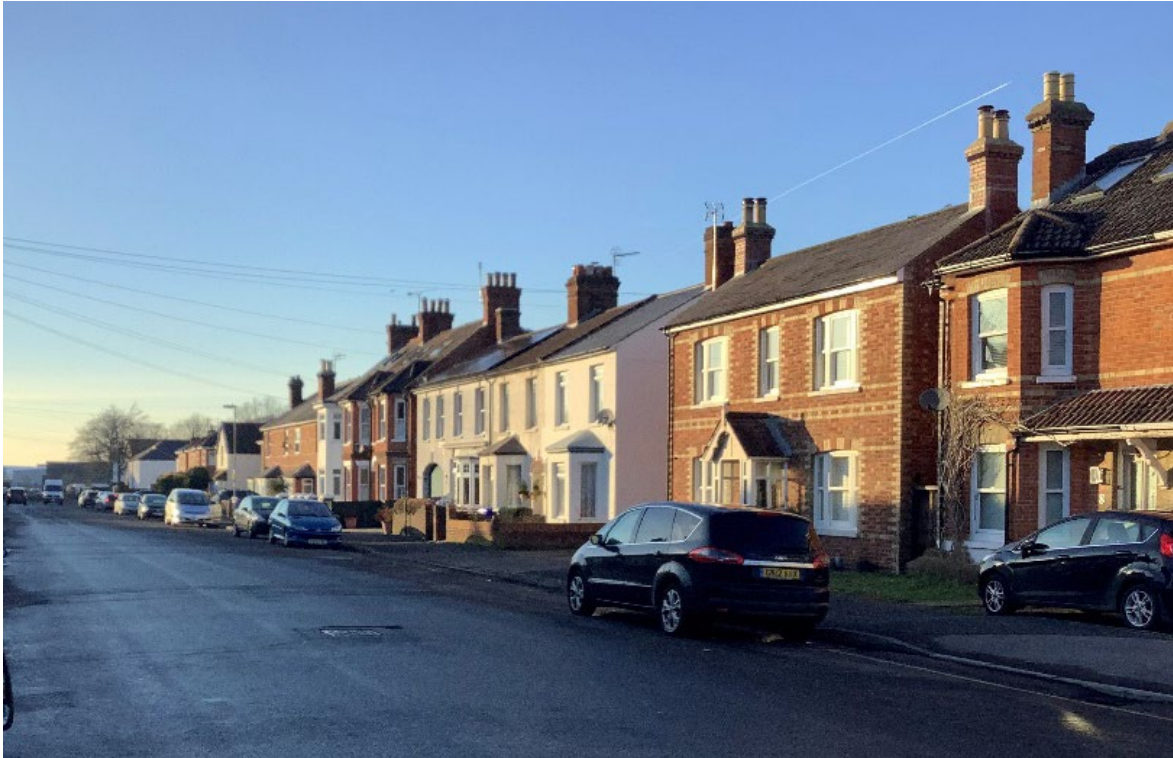
Cross Street North Side
